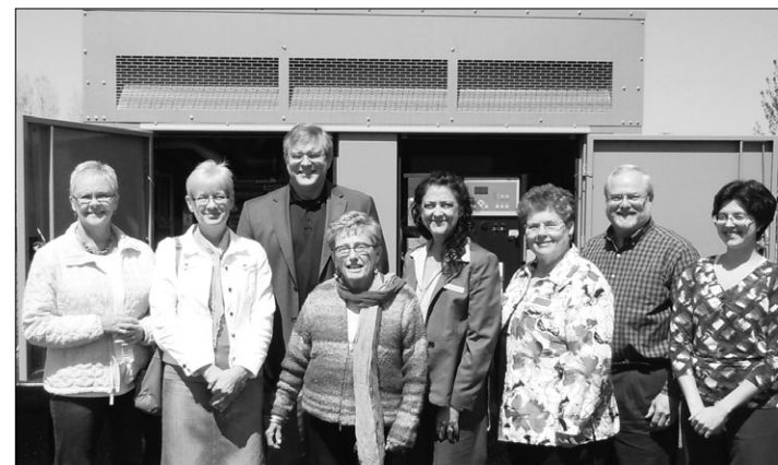
Some of the donors who made the new generator possible
